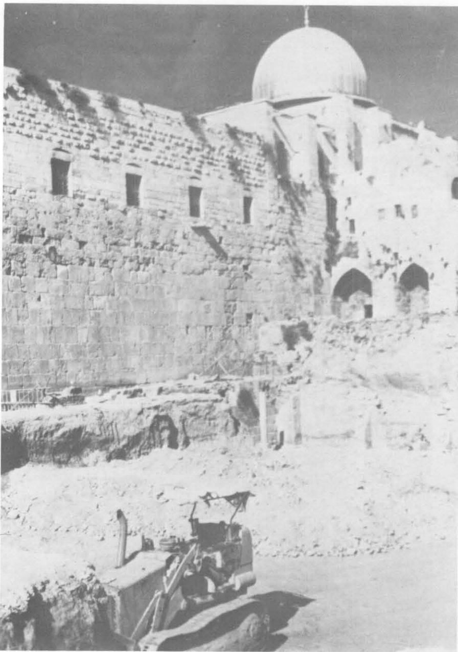
Bulldozing operation at the southern wall of the Haram esh-Sharif
